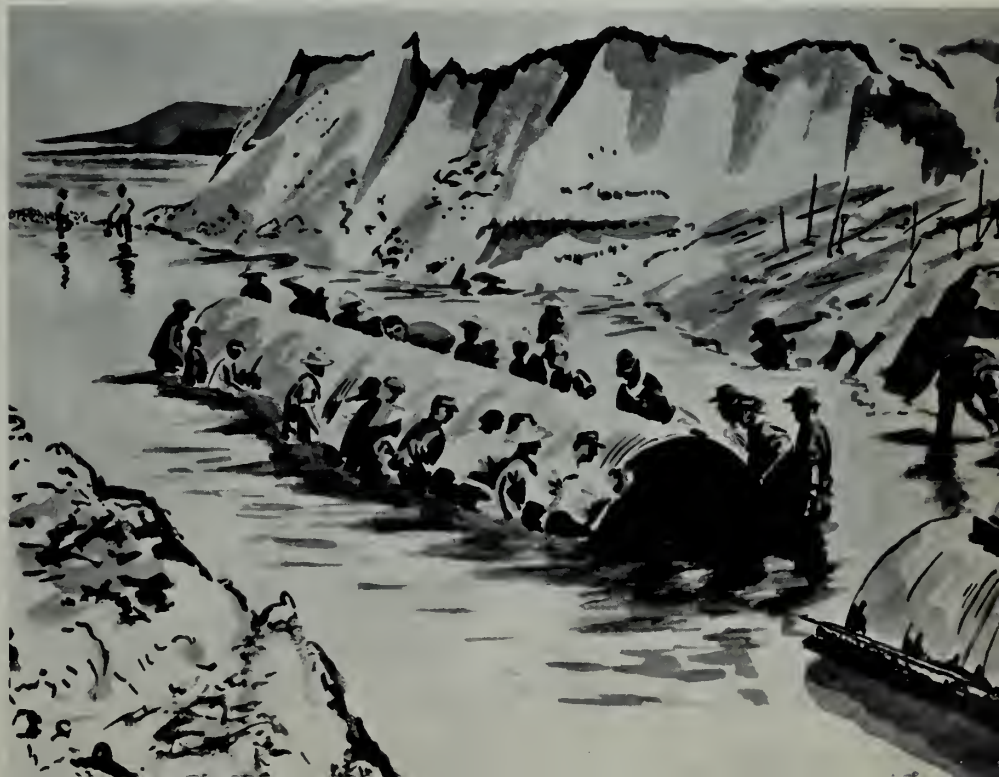
Culverts keep low areas dry, prevent roads from being washed out by monsoons. Drawing by SP4 Robert S. Schipp.
